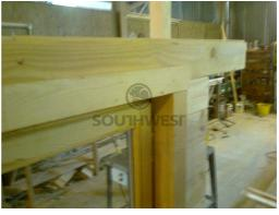
3. Screws can be place in the bottom wall log if required as this wall log will not settle any further.
