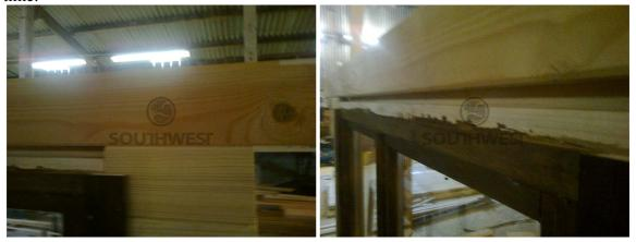
2. The window and door fascias are fitted all round the windows/doors inside and outside. Fix fascia boards to window frame only, not wall logs. The wall logs must be free to move.
