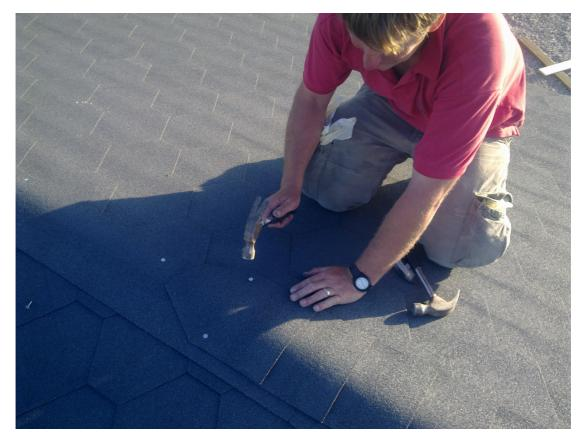
For the ridge overlap the top layer of shingles on both sides. The ridge tile is cut down from a standard shingle using a Stanley knife. Install as picture.
